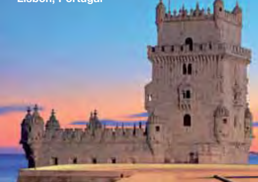
Belem Tower Lisbon, Portugal
